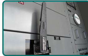
Metered Switchboard
