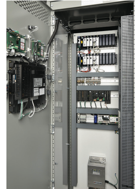
Master Control with Redundant PLC's
