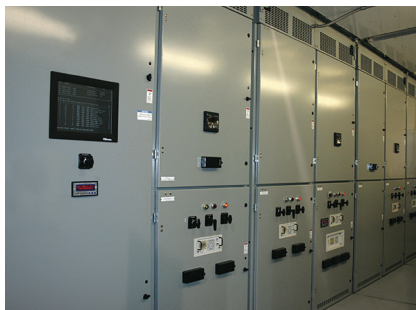
Medium Voltage Paralleling Switchgear
